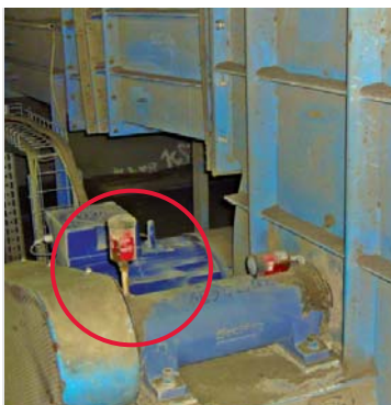
Fan drive shaft lubrication (2 points)
