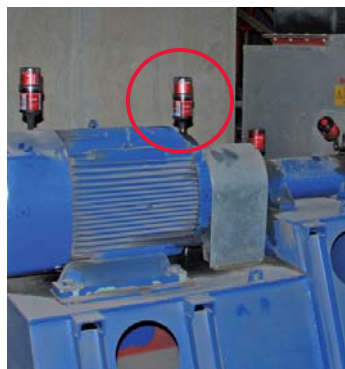
Drive motor lubrication (2 points)
