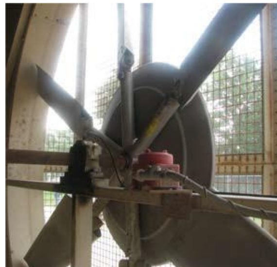
Tubing from PRO MP-6 being run to end bearing on gas compression engine cooling fan.
