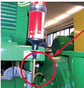
Gland lubrication (1 point)
