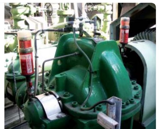
Lubrication system: 2 perma STAR VARIO 250 cm 3 each
